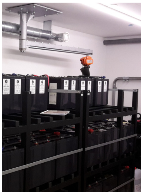
Figur 7: Batterilager, 144kWh bly-kiselgel
